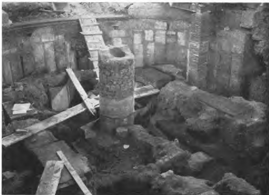
Fig. 59 — S. Lorenzo f.l.m. Excavations 1947-49. L-chamber, cataract and apse K during construction of shelter, 1950 (Photo: Soprintendenza ai monumenti).
